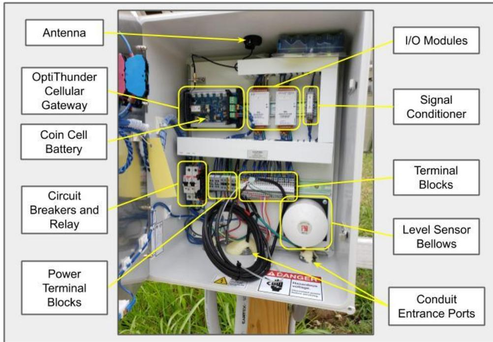
**Figure 4:** Opti control panel annotated with major components
