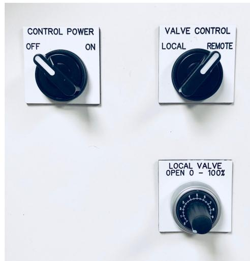
**Figure 3:** Opti Control Panel swing door controls
